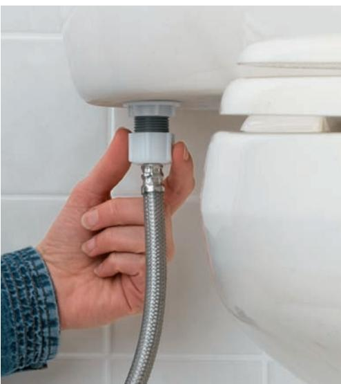
**12** Hook up the water supply by connecting the supply tube to the threaded fill valve with the coupling nut provided. Turn on the water and test for leaks.
