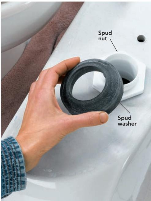
**6** Attach the toilet tank. Some tanks come with a flush valve and a fill valve preinstalled, but if yours does not, insert the flush valve through the tank opening and tighten a spud nut over the threaded end of the valve. Place a foam spud washer on top of the spud nut.
