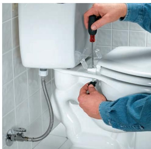
**13** Attach the toilet seat by threading the plastic or brass bolts provided with the seat through the openings on the back of the rim and attaching nuts.
