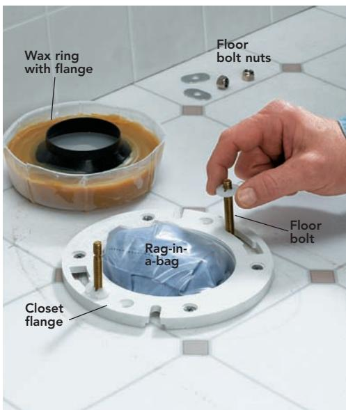
**4** Remove the rag-in-a-bag from the drain opening and put new all-brass toilet bolts into the slots on the closet flange at 3 and 9 o'clock and rotate each  $\frac{1}{4}$  turn so the elongated heads cannot be withdrawn. Put the plastic keepers or extra washers and nuts on the bolts to secure them to the flange. Unwrap the wax ring and position it over the flange so it looks like the one in the cross section photo at the top of this page.
