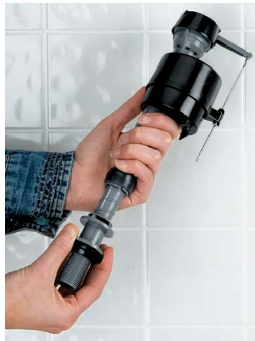
**7** If necessary, adjust the fill valve as noted in the directions (also see pages 54 to 57).
