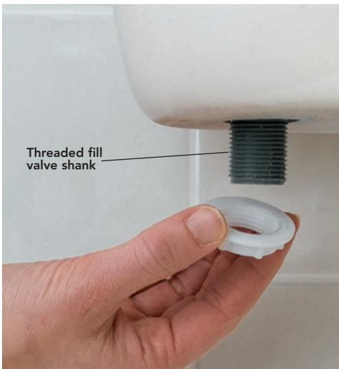
**8** Position the valve in the tank. Push down on the valve shank (not the top) while hand-tightening the locknut onto the threaded valve shank (thread the nut on the exterior side of tank). Hand-tighten only.
