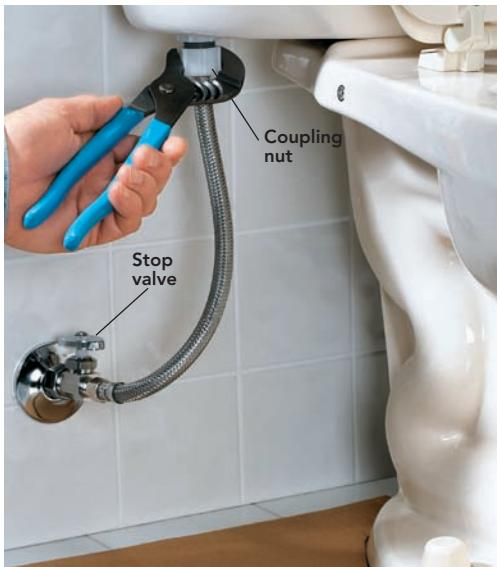
**1** Remove the old toilet. First, turn off the water at the stop valve (see page 18 if you have trouble). Flush the toilet holding the handle down for a long flush, and sponge out the tank. Unthread the coupling nut for the water supply below the tank using channel-type pliers if needed. **TIP:** If you have a wet vac, use this here and in step three to clear any remaining water out of the tank and bowl.
