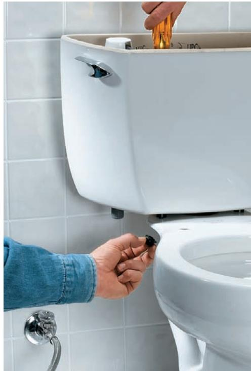
**11** You may stabilize the bolts with a large slotted screwdriver from inside the tank, but tighten the nuts, not the bolts. You may press down a little on a side, the front, or the rear of the tank to level it as you tighten the nuts by hand. Do not overtighten and crack the tank. The tank should be level and stable when you're done.
