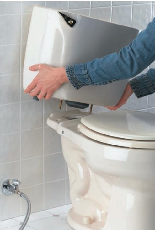
**10** Position the tank on the bowl, spud washer on opening, bolts through bolt holes. Put a rubber washer followed by a brass washer and a wing nut on each bolt and tighten these up evenly.
