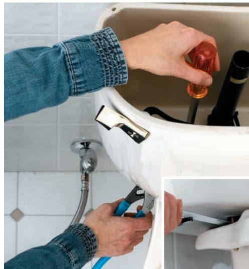
**2** Grip each tank bolt nut with a box wrench or pliers and loosen it as you stabilize each tank bolt from inside the tank with a large slotted screwdriver. If the nuts are stuck, apply penetrating oil to the nut and let it sit before trying to remove them again. You may also cut the tank bolts between the tank and the bowl with an open-ended hacksaw (inset). Remove and discard the tank.
